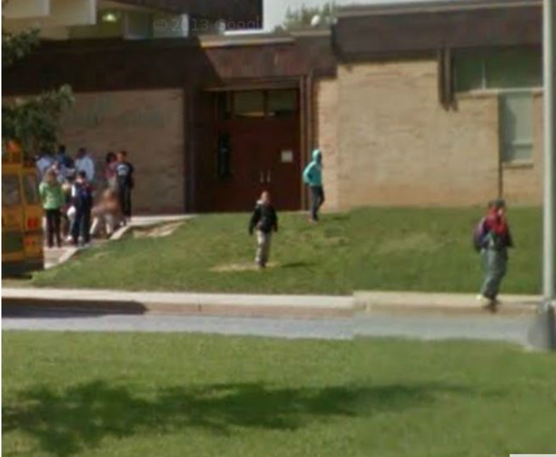
Middle School 1970. Less glazing / Glass in front. A vehicle still can drive right up.
