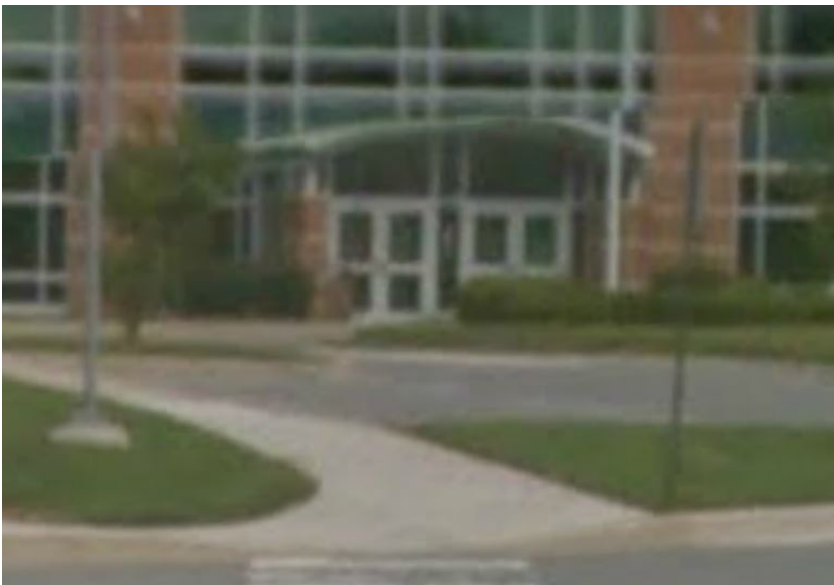
High School built 2003. No Added Security Features. Too much glazing/ windows. No protection from vehicles.
