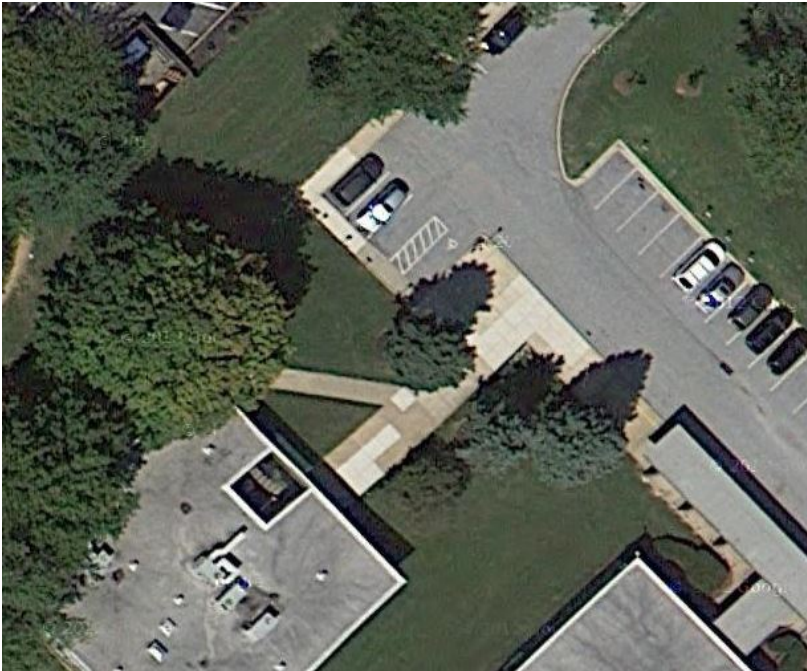
Same High School overhead photo show no devices to stop a vehicle.
